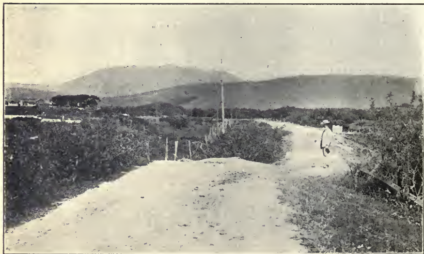
What the great earthquake of 1906 did to the road near Pt. Reyes. The road was broken and the parts shoved past each other twelve feet.
